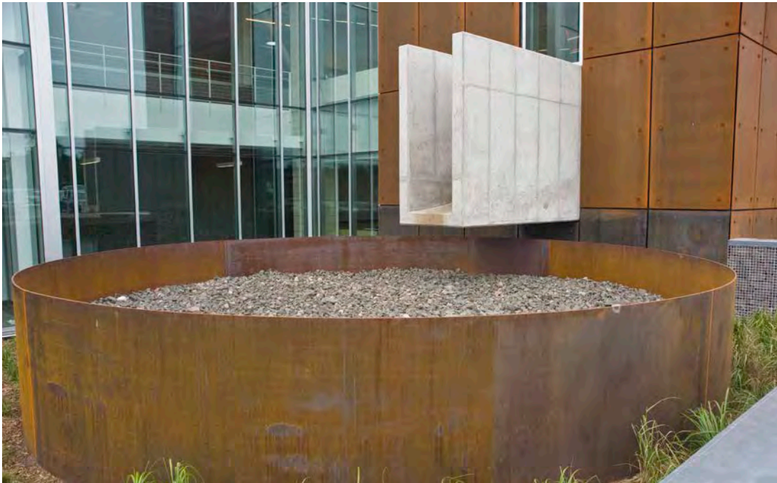
Left Above: HCAMS outdoor landscape Left Below: Swenson Civil Engineering stormwater management
